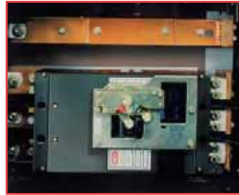
MCCB Rotary Handle Mechanism
